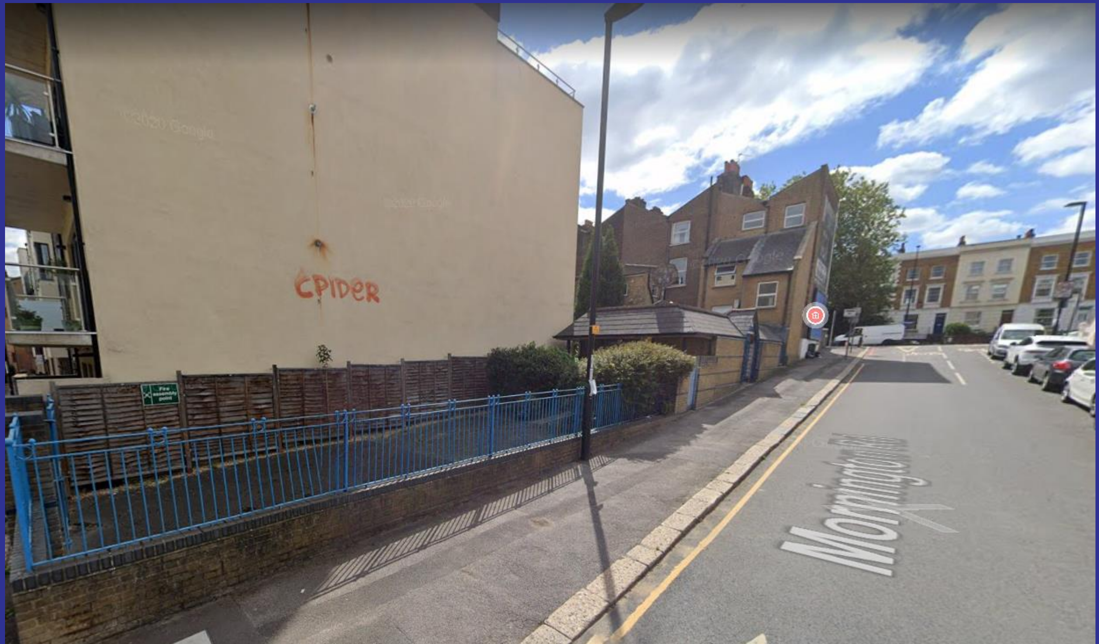
Rear and side of the site
